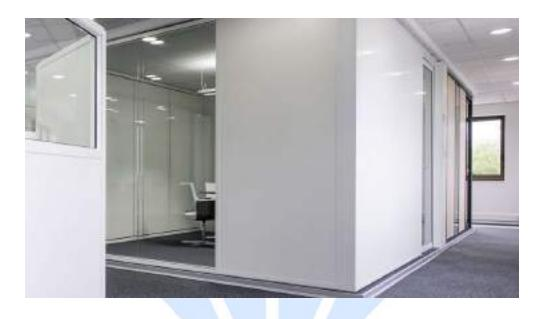
A high performance lightweight interior wall system consisting of a GI steel frame, encased in gypsum plasterboards on either side attached with self-drilling drywall screws. The joints are then taped and finished with gypsum jointing compounds.
