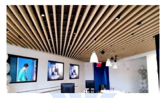
Linear Baffles is an attractive, linear ceiling system that screens the open plenum beautifully. It has Clean crisp detailing and detachable suspension with fully adjustable spacing. It is a Robust, engineered system that is quick and easy to install.
