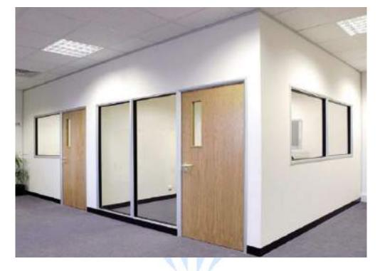
Gypsum drywall is an effective building a material because gypsum is very fire-resistant. The gypsum molecule contains within it two water molecules and one calcium sulphate. Gypsum creates a more rigid plaster than lime and does not require a fiber additive like animal hair as lime plaster does.
