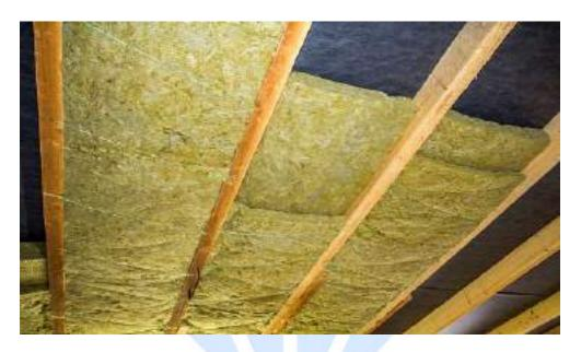
Rockwool insulation refers to a type of insulation that is made from actual rocks and minerals. It also goes by the names of stone wool insulation, mineral wool insulation, or slag wool insulation. A wide range of products can be made from Rockwool, due to its excellent ability to block sound and heat. Rockwool insulation is commonly used in building construction, industrial plants, and in automotive applications.
