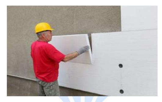
Thermocol or EPS sheets are in fact an excellent thermal insulator for the Indian climate. They are lightweight and affordable (making them easy to install), with a high insulation value. Thermal insulation empowers consistency in room temperature by keeping the room cooler in summer and hotter in winter all things considered. It is energy saving as the transfer of heat from inside to outside and the other way around is restricted.
